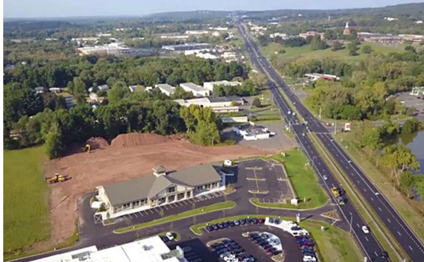
Turnpike Ridge construction Source: Hartfordbusiness.com
