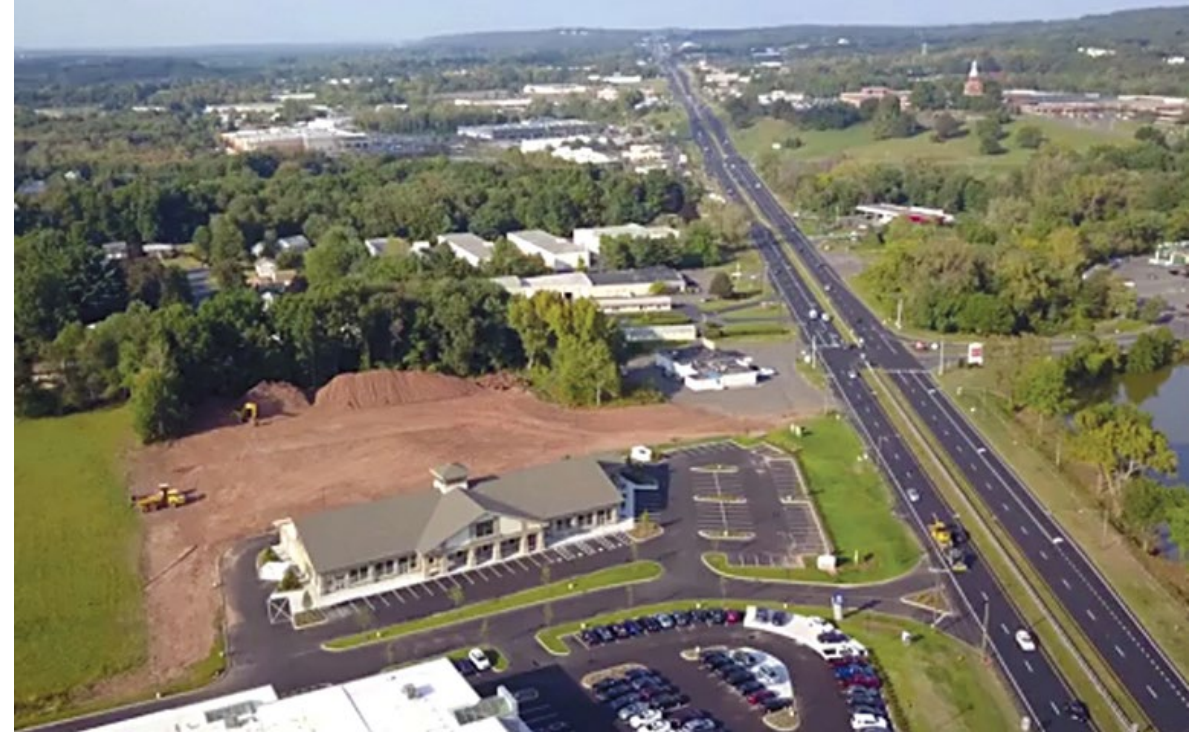
Turnpike Ridge construction Source: Hartfordbusiness.com
