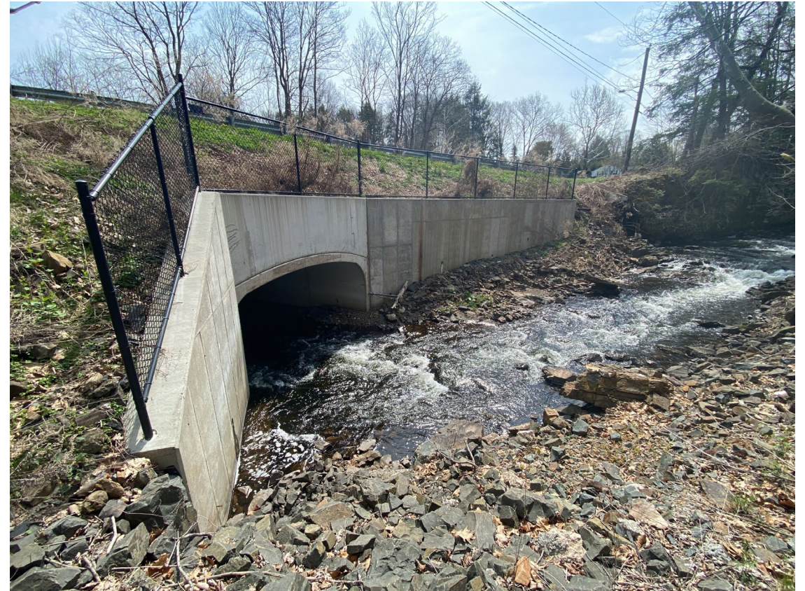
New High Street Bridge
