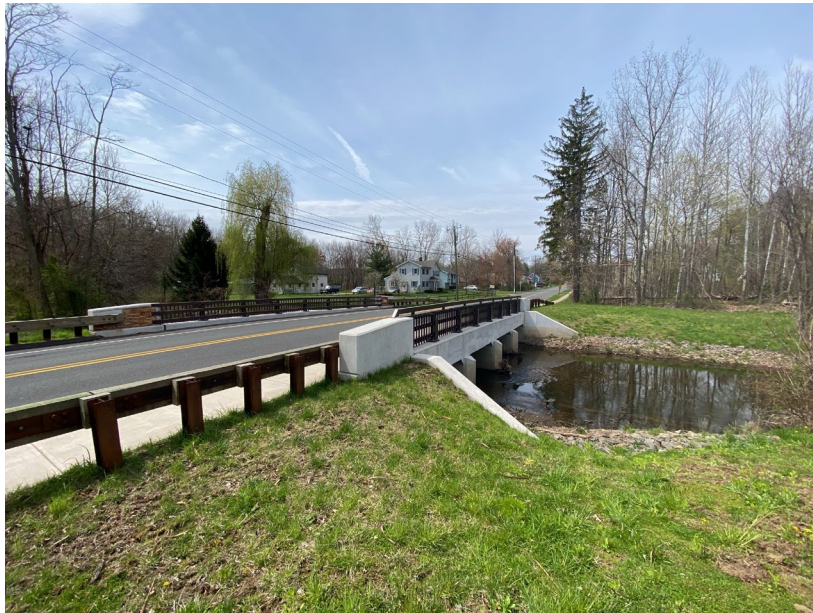
Recently reconstructed Burnham Street Bridge
