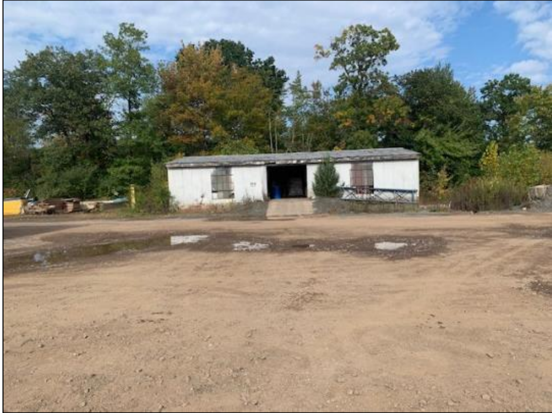
Exhibit 3: Existing Shed to be Demolished
