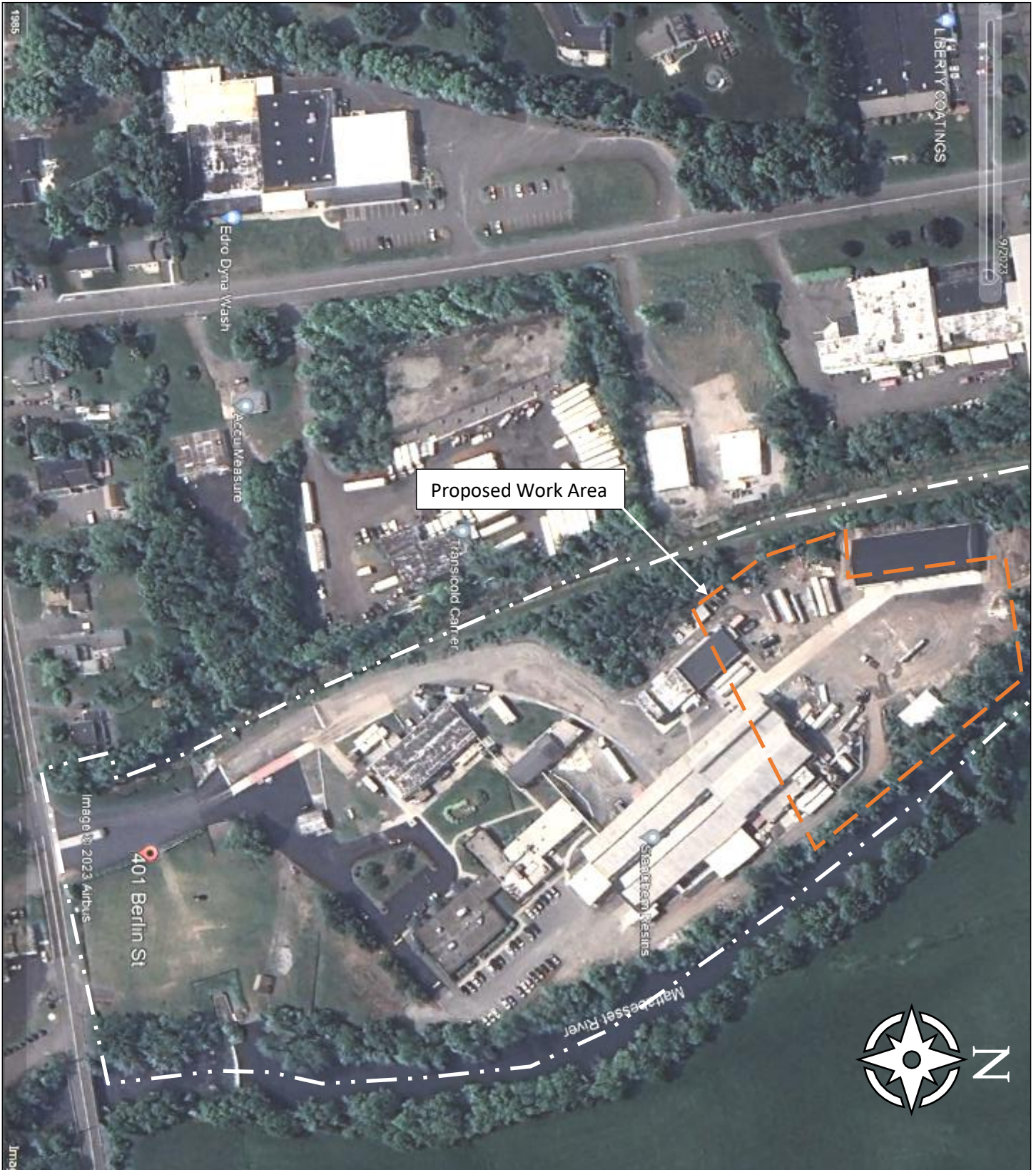
Exhibit 1: Overall Existing Site Photo
