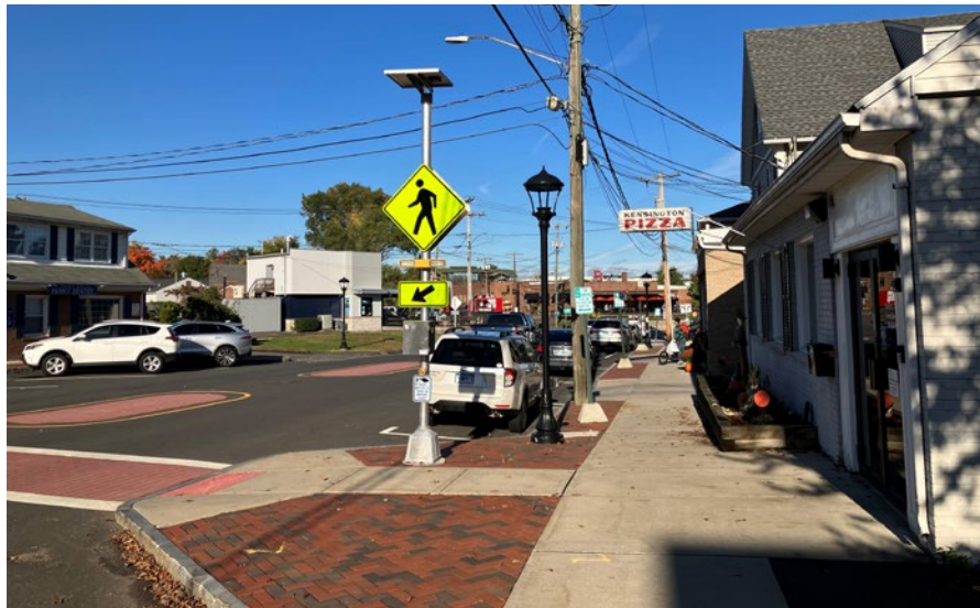
Kensington Center Streetscape Enhancements
