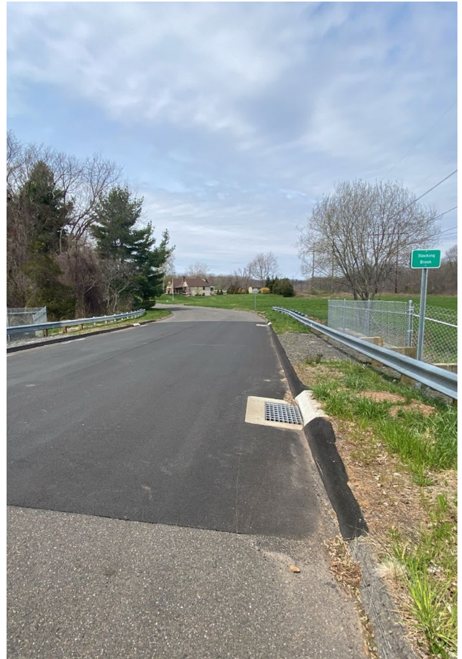
Recently improved segment of Heritage Drive Image Source: Town of Berlin
