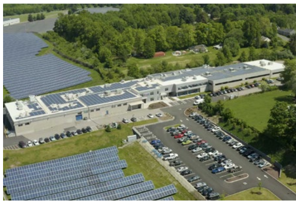
Recently Expanded TOMZ Corporation Headquarters Source: TOMZ Corporation
